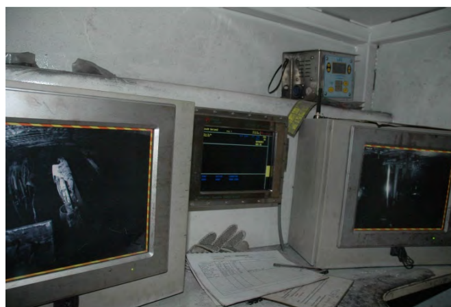
Figure 4 – Example Control Room
